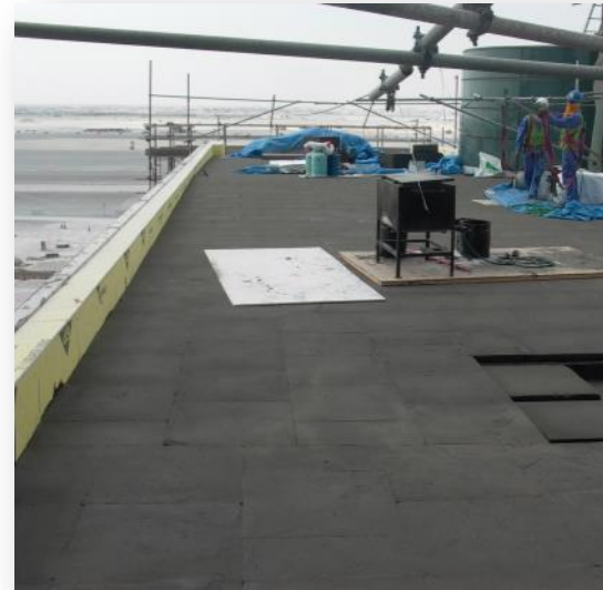
Job site picture during application
