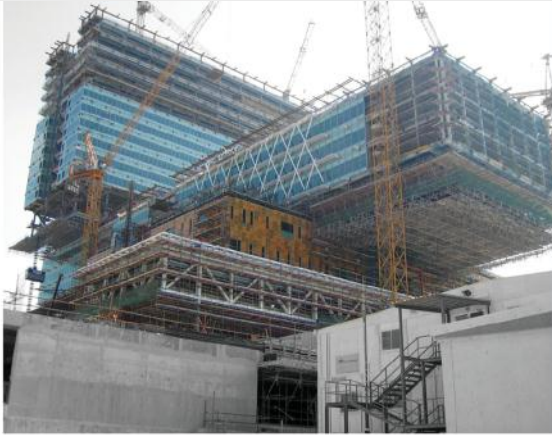
Flat roof, Terraces
