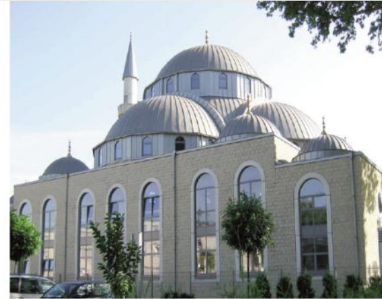
Mosque New building
